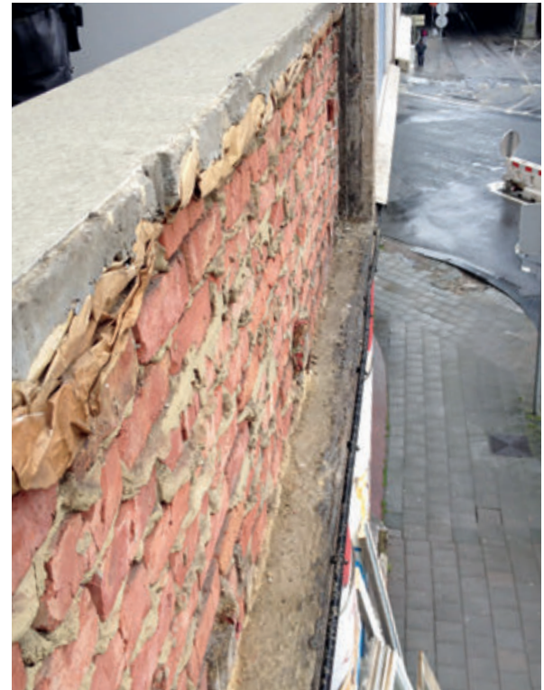
brick wall behind the sandwich panel (exposed during renovation, 2016)
