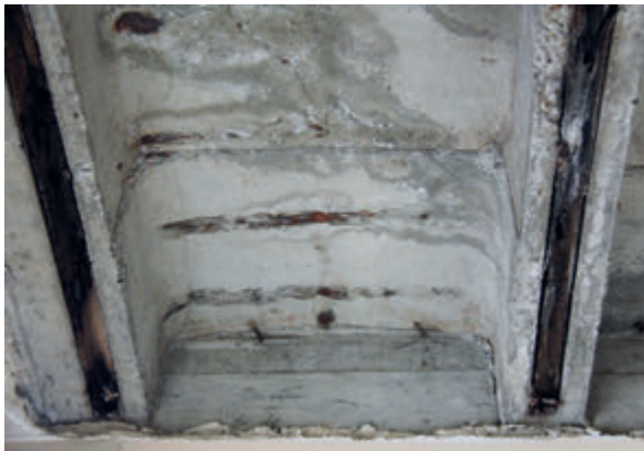
the concrete ribbed floor cast in situ, seen from below (2016)
